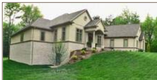
The exterior of an Evansville home built with Insulated Concrete Forms by Cravens Construction Co.
